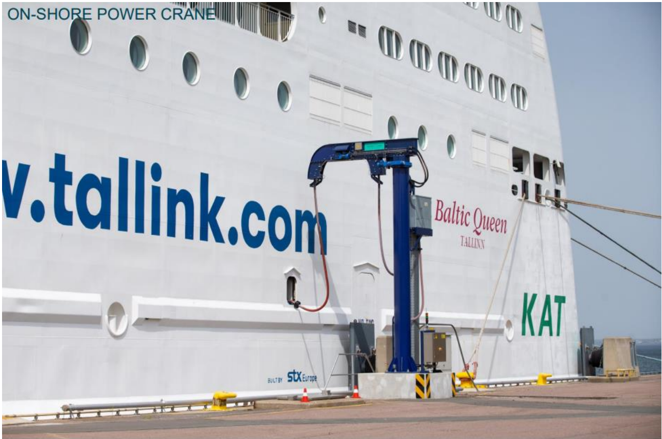
Figure 19 TWIN-Port III - On-Shore Power Crane
